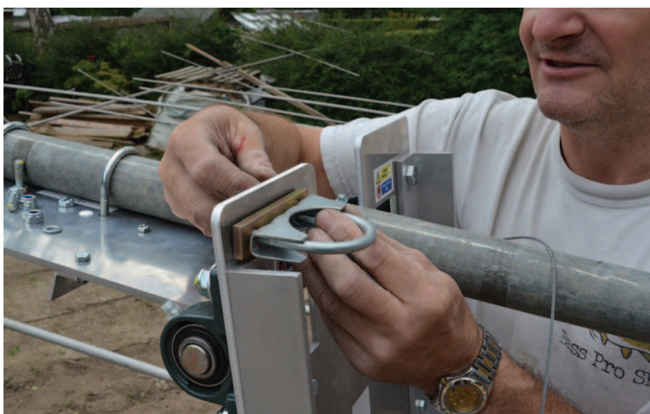
Chris, GODWV mounts the clamps for the boom truss support.
