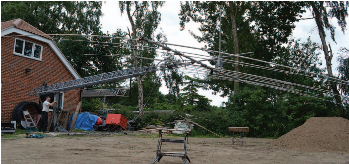
As the tower is cranked up the antenna automatically remains horizontal.
